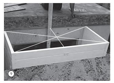
Before back filling, each section should be braced both in the corners and in the center. Clean stone provides the least pressure on the walls. Even though the walls are reinforced with a galvanized steel channel, care should be used in back filling to avoid causing distortion.
