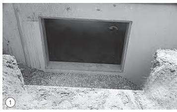
Properly prepared, a well site is over-cut 4"- 6" This will leave sufficient area to be "back filled" with clean ¾" stone after the installation is complete. Before installing the first well section, put 4" of clean ¾" stone below the window.
