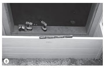
Drive screws into top holes of side panels. Level. Screw remaining screws into the pre-drilled holes.
