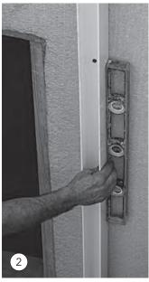
Mark the wall for U-channels according to the width of the window well. Make sure it is evenly spaced with the window in the center. Using Tapcon™ screws, attach first U-channel at desired height with top of channel 4" above final grade. Make sure it is plumb before attaching.
