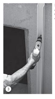
Level accross to find position of second U-channel height. Check for plumb. Attach to wall.
