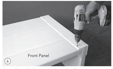
Set well upside down onto the sidewalls and secure corner connector using pilot holes and supplied #14 ¾" white screws. Note: Keep sidewalls and front panel flush in the corner connector channel before securing with screws.
