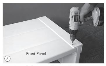
Set well upside down onto the sidewalls and secure corner connector using pilot holes and supplied #14 ¾" white screws. Note: Keep sidewalls and front panel flush in the corner connector channel before securing with screws.
