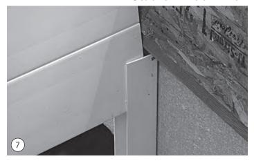
Carefully transfer the assembled well section to the mounting channel and slide it into place to arrow in channel. Drive in top screws.
