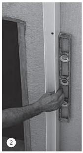
Mark the wall for U-channels according to the width of the window well. Make sure it is evenly spaced with the window in the center. Using Tapcon™ screws, attach first U-channel at desired height with top of channel 4" above final grade. Make sure it is plumb before attaching.
