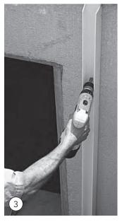
Level accross to find position of second U-channel height. Check for plumb. Attach to wall. Using a silicone caulking, place a bead of caulking along side of U-channel at the wall.
