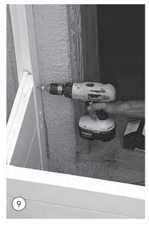
Repeat steps 5, 6, 7, and 9 to assemble the next course, and then position and secure it. Use a bead of caulking between each course.
