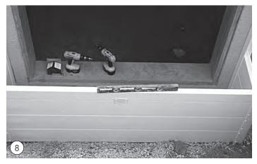
Place a level on a side panel. Keeping front slightly high, drive two screws into each plank in the wall, starting at the bottom. Note: Front panel needs to be perfectly level. Drive screws into the other side panel.
